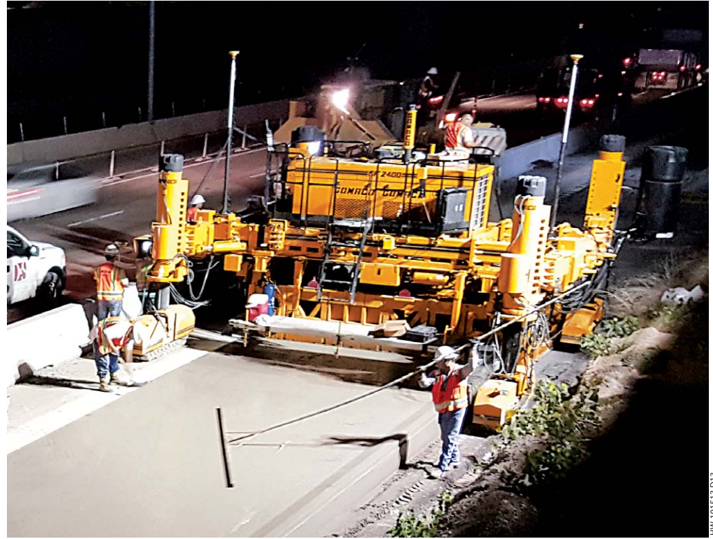
The GOMACO four-track GP-2400 scabs on a single lane with an integral curb on the right side during a night pour using 3D machine guidance.
