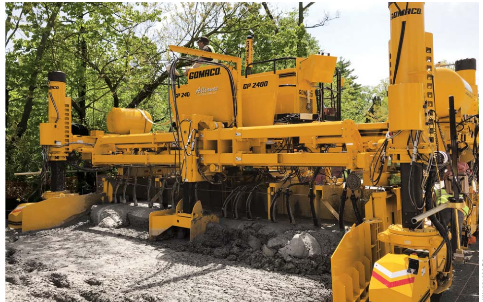
Existing trees created tight-clearance conditions for this four-track GP-2400. The paver is equipped with a 5000 series paving mold and a spreader plow to level the concrete ahead of the slipform paver.
