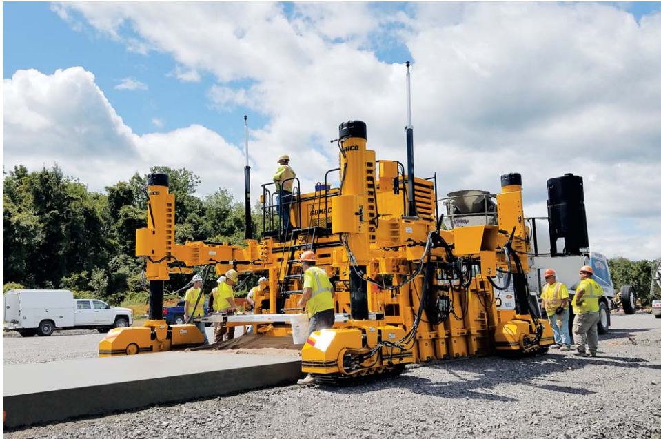
Mainline highway paving is being performed with ease using this four-track GP-2400 equipped with 3D machine guidance.
