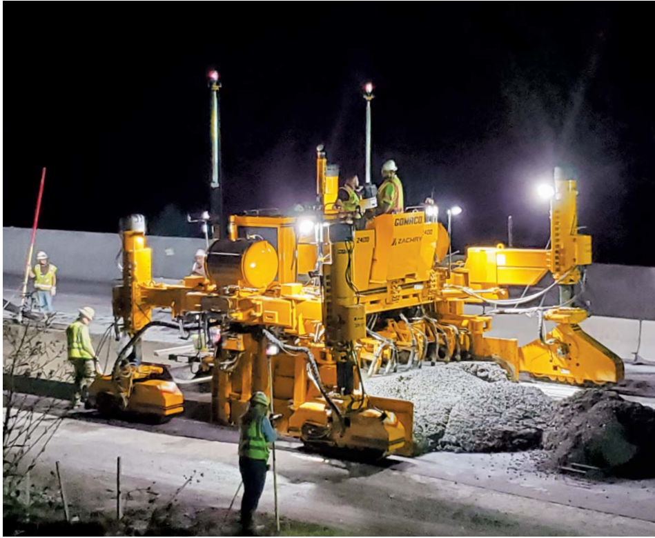
A GOMACO four-track GP-2400 with optional rotary-sensored slew drives slipforms a highway using 3D machine guidance. The left side is using high-rise tracks that are only six inches (152 mm) wide to achieve minimum clearance.
