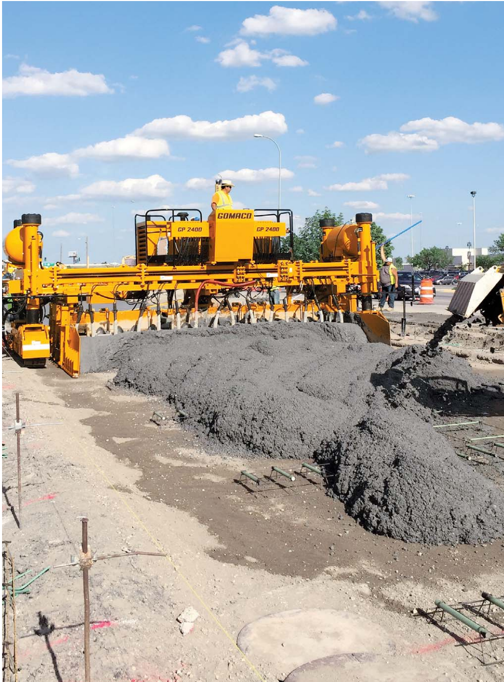
The GOMACO RTP-500 places concrete over dowel baskets in front of a two-track GP-2400 slipforming a new city street.
